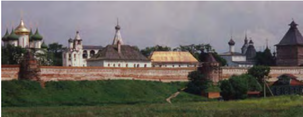
A view of the Susdal Monastery from outside the perimeter walls.
