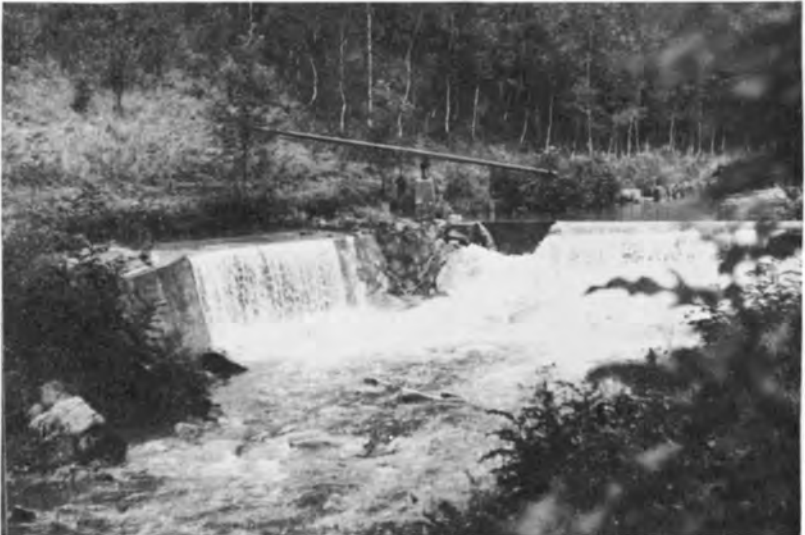
Pilgram Marpeck built channel dams to float Black Forest lumber down the Kinzig River.
